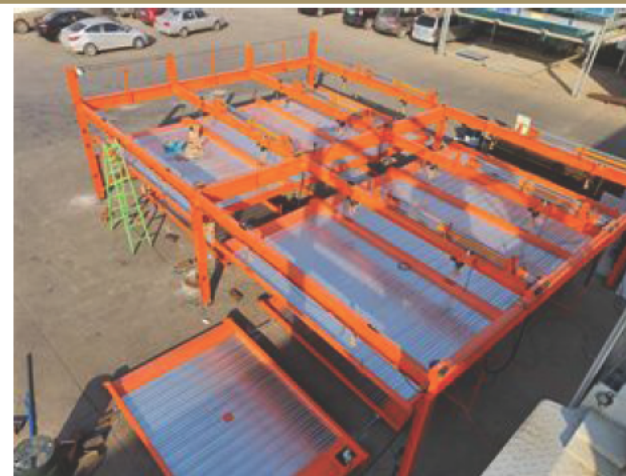
Construction Progress | Car Stacker Mock Up
